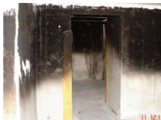
Figure C-7: Interior View of Burn Prop
