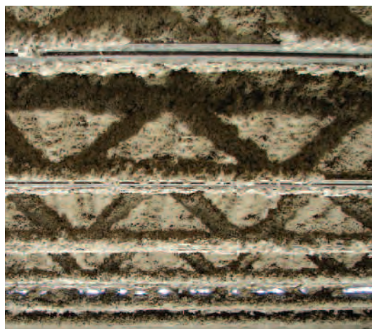
Figure C-4: Fireproofing added to structural steel
